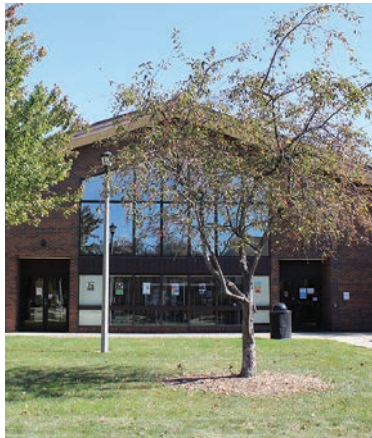
Douglass Community Center
