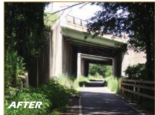
AFTER: Trail underpass installed beneath a highway to connect two segments of a trail.
