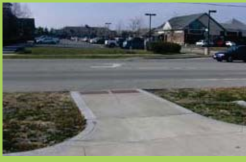
A potential crossing point for the "C" connector near Village Office Place (a private street at the north end of Hallbeck Park)
