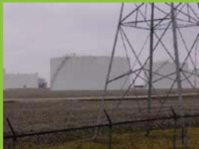
Marathon Oil storage facility
