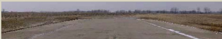
Olympian Drive looking east where the extension would cross the CN Railroad
