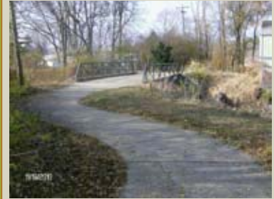
Segment "A" would connect with the existing O'Malley's Alley Trail east of the Duncan Road.
