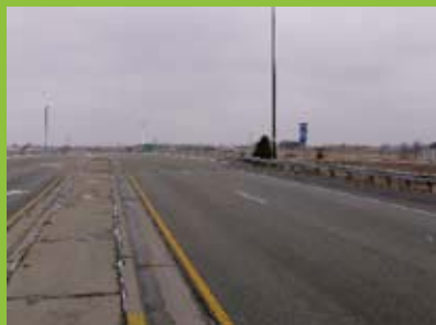
Interstate 57 and Olympian Drive overpass
