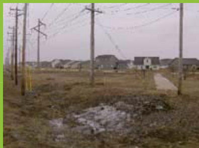
Drainage ditch at Prospect Avenue and Olympian Drive
