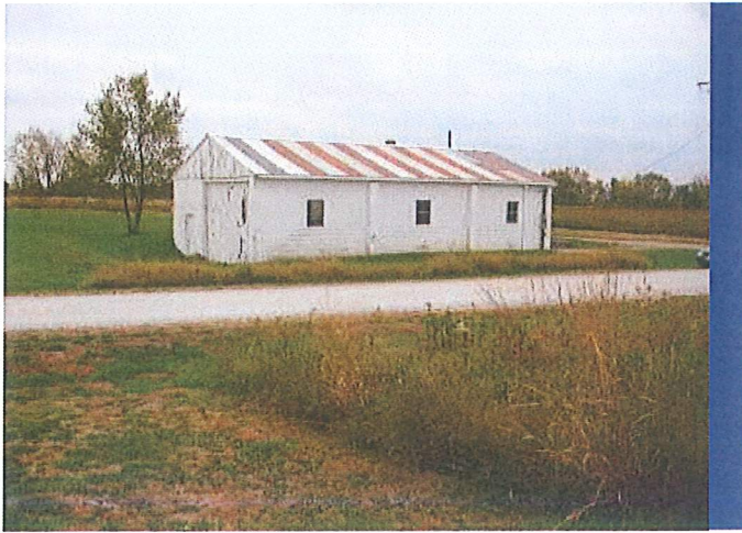
Existing storage structure - currently used by the Champaign County Radio Control Club (looking southeast).
