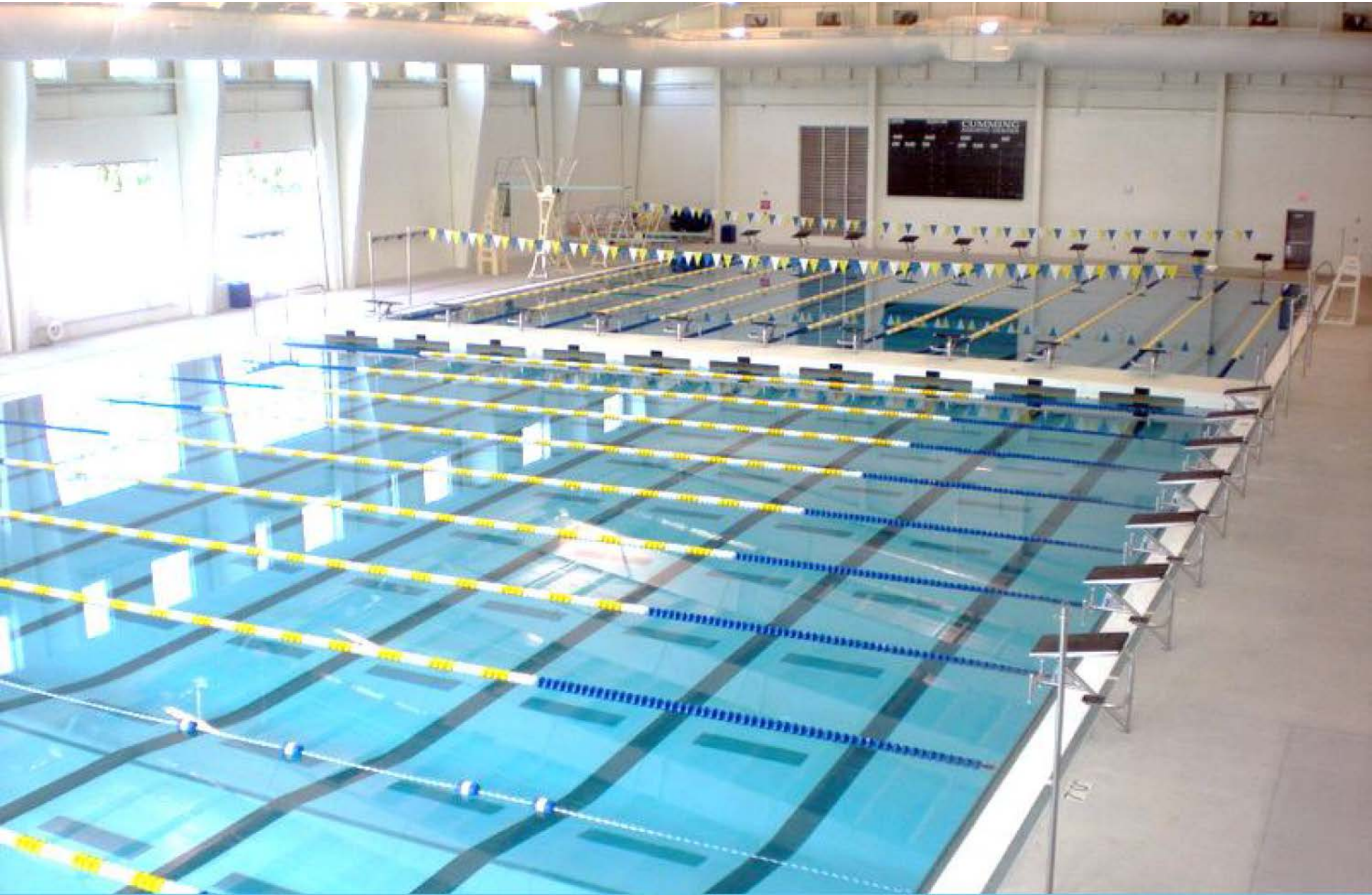
SPALDING AQUATIC CENTER 50 M. LAP POOL
