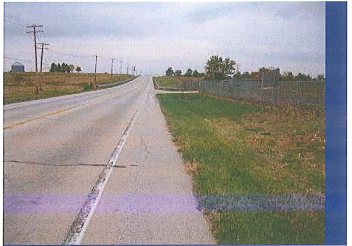
Entrance/exit to site looking west along Route 150.
