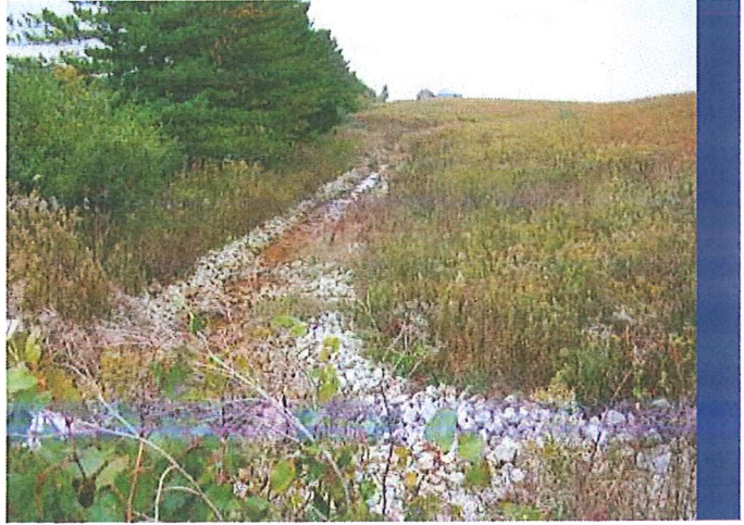
Drainage ditch along south-east side of property line (looking south).
