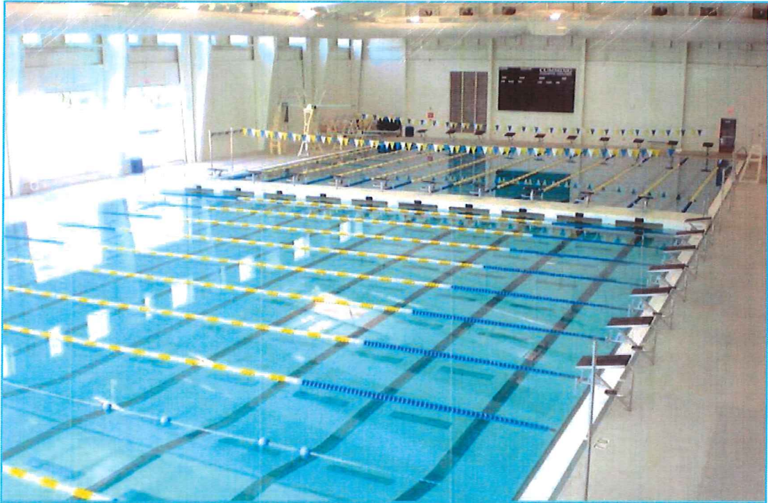
SPALDING AQUATIC CENTER 50 M. LAP POOL
