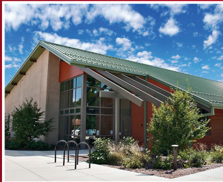
Planning & Operations Facility, Urbana Park District
