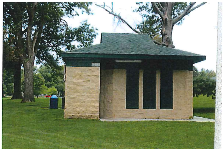
Hessel Park Bathrooms
