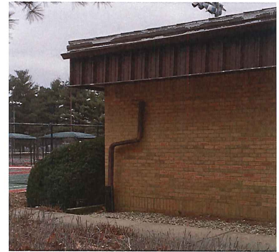
Disconnected downspout
