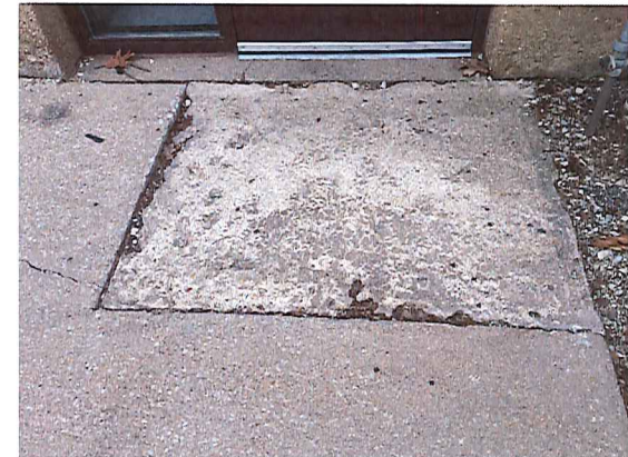
Pavement near exit door
