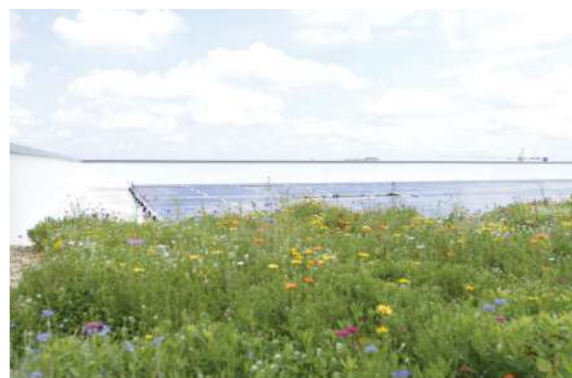
Green Roof Systems With Native Plantings
