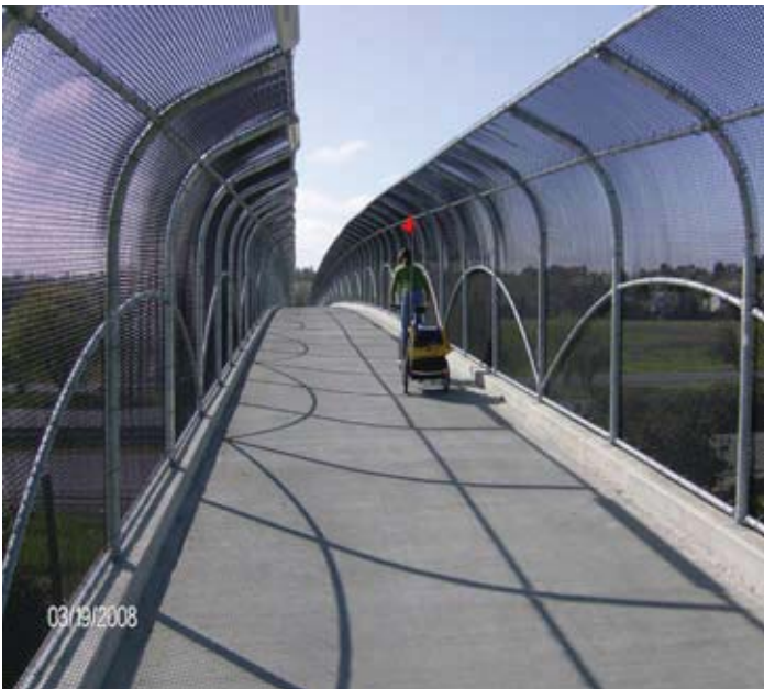
An example of a bicycle/pedestrian overpass bridge.
