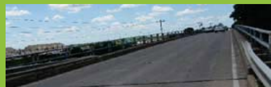
Limited space on the existing bridge over Interstate 57
