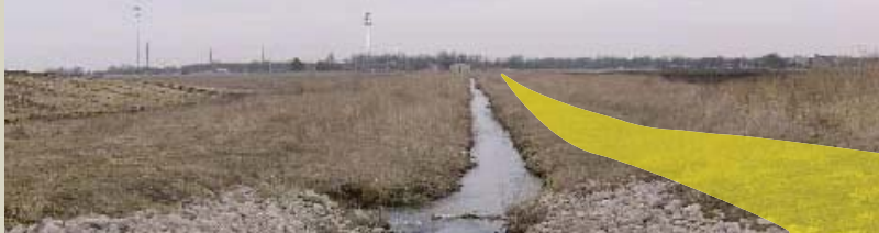
Phinney Branch looking north from its connection with Curtis Road.
