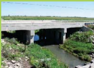
The Kaskaskia River and Route 10 / Springfield Avenue
