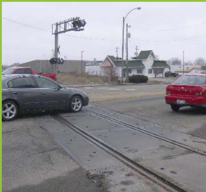
The Wabash Railroad crossing at Prospect Avenue
