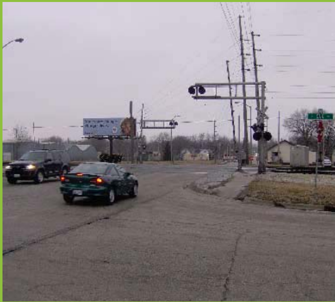
Bradley Avenue at the CN Railroad tracks. The Boneyard Greenway would need to cross the tracks at this location.
