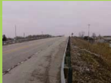
U.S. Route 150 as it crosses Interstate 57
