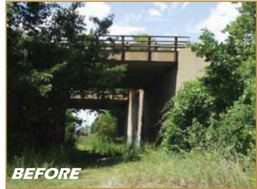
BEFORE BEFORE: Trail pavement needed to turn into a multi-use trail.
