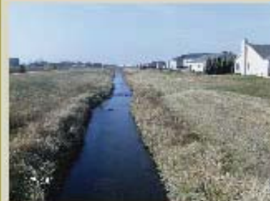
The Lower Copper Slough looking west from the existing Pipeline Trail.
