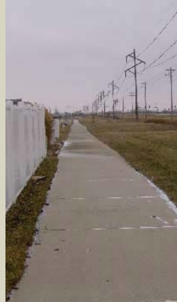
Existing trail segment along Olympian Drive
