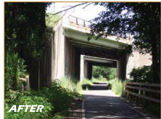
AFTER: Trail underpass installed beneath a highway to connect two segments of a trail.
