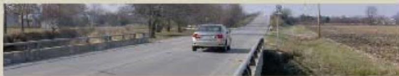
Kirby Avenue heading west towards the bridge over Interstate 57
