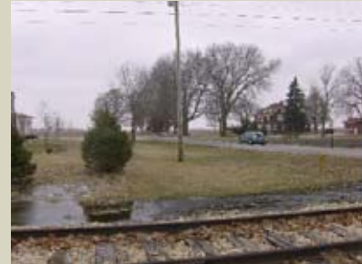
Rising Road connection at the Wabash Railtrail
