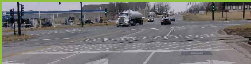
The West Springfield Avenue Railtrail will need to cross this intersection at Staley Road
