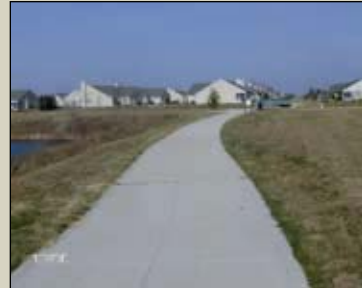
Looking north along the Pipeline Trail from Windsor Road.
