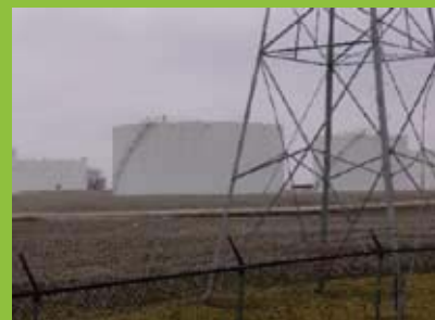
Marathon Oil storage facility
