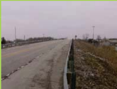
U.S. Route 150 as it crosses Interstate 57
