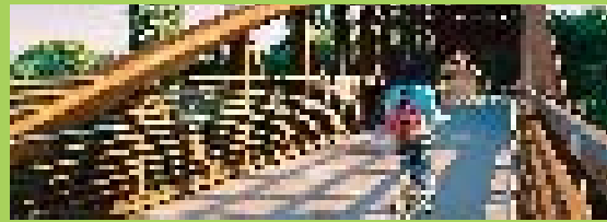
An example of a bicycle / pedestrian only overpass
