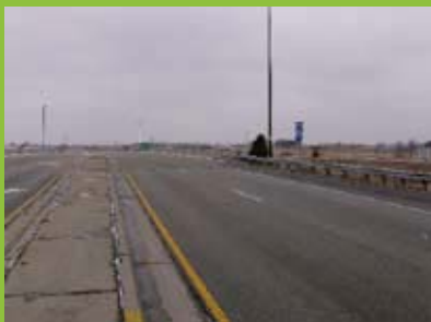
Interstate 57 and Olympian Drive overpass
