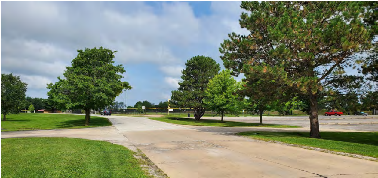
Figure 3: Parkland Way Concrete Pavement Surface
