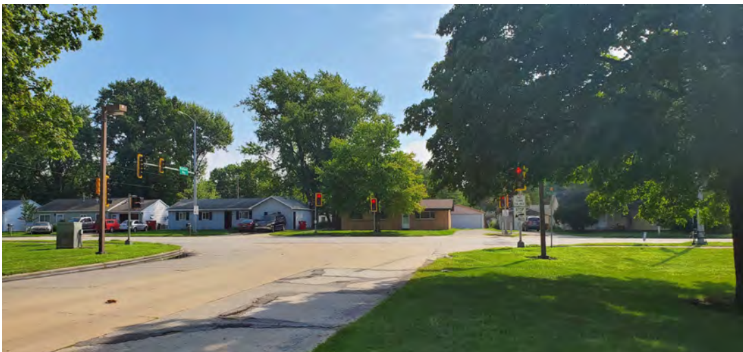
Figure 5: Parkland Way eastbound at Mattis Avenue
